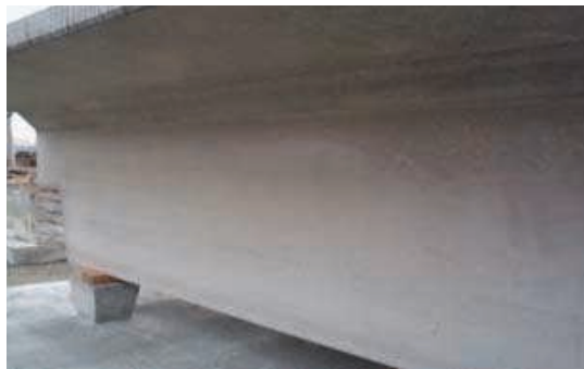
Self-Consolidating Concrete provided a consistent, durable and high-quality finish.
