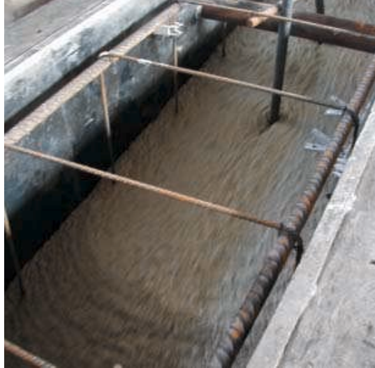
The use of Self-Consolidating Concrete from Grace shortened construction time and reduced the manpower required for the job.
