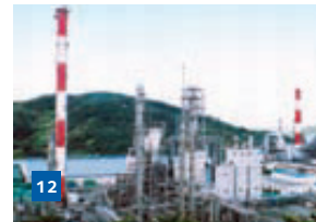
10 Barbados Light & Power Plant | Barbados 11 Braidwood | Braidwood, IL, USA 12 GS Caltex Facilities | Yeochon, S. Korea
