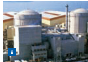
7 Vought Aircraft Ind. - Boeing Aircraft | Charleston, SC, USA 8 Hyundai Petrochemical Plant | Daesan, S. Korea 9 Daya Bay Nuclear Power Plant | Guangdong, China
