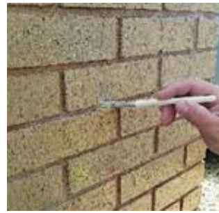
Brushing in raked mortar joints
