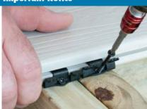
Butt joints should be attached using two deck clips for additional strength. Using two clips at but joints will allow for any shrinkage, swelling or other movement that may occur. The second clip may be added by scabbing a runner board to the joist and attaching a deck clip.
