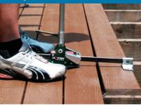
Begin the next board by sliding the board onto the double leg side of the deck clips. Make sure the new deck board is secured tightly against the deck clips for consistent gapping. Repeat steps 2 and 3.
