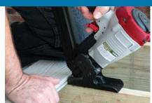
Fasten Deckmaster clips to the joist using the deck screws provided. Slide the screw into the deck clip guide hole and secure at a 45° angle into the joist.
