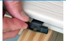
Insert Deckmaster clips into the groove in the deck board at each joist.
