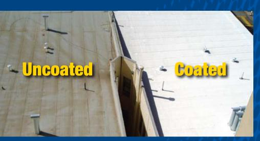
ENERGY STAR compliant Henry white roof coatings can significantly reduce the energy costs required to keep a building or home cool.
