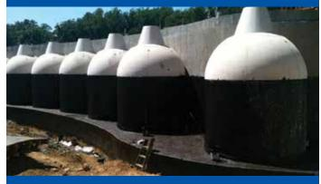
Henry<sup>®</sup> CM100 waterproofing membrane is ideal for a variety of applications, including vertical and horizontal as well as complex geometries.
