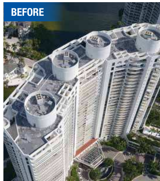
Photos courtesy of Florida Quality Roofing
