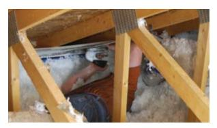
Stapled in place sheet applied or foil radiant barriers can be difficult and time-consuming to install in existing home attics.
