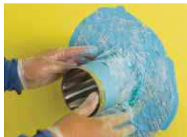
Pipes and Other Through Wall Penetrations
