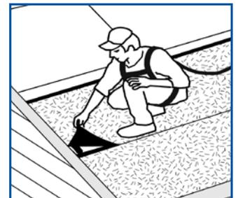
Seal at rake and set in place. Apply pressure at laps (image 14).
