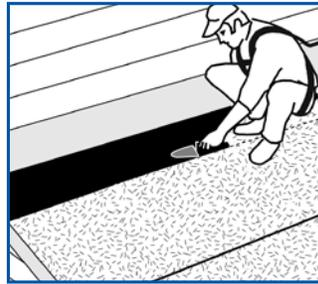
Spread sealant over surface evenly with trowel. Allow to dry for 1 hour minimum.
