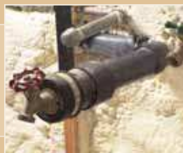
SEALS PIPES AND THROUGH-THE-WALL PLUMBING PENETRATIONS.
