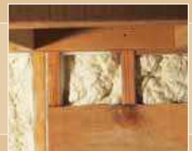
SELF-ADHESIVE SPRAY SEALS SMALL, TIGHT SPACES, UNDERSIDE OF ROOF SHEATHING AND FLOOR BOARDS.
