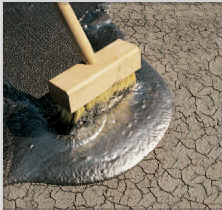
**Uses:** Coat smooth surfaced built-up roofing, modified bitumen membranes, roll roofing and metal roofs.
