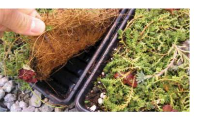
A coconut fiber mat is at the bottom of the soil profile, holding the plants together, and allowing easy handling. Tiles are simply laid down on bare soil.
