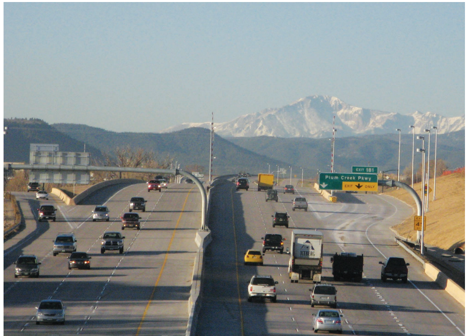
C1157 Blended Cement paved I-25
