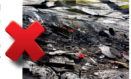
▲ Traditional asphalt roofing waste
