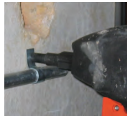
12HSMPO34 clip assembly used to secure conduit
