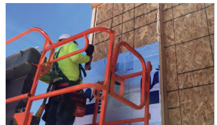
Behind cladding over wood stud walls
