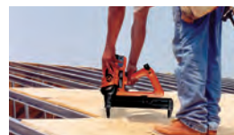
Plywood attachment—using TrakFast plywood to steel pin
