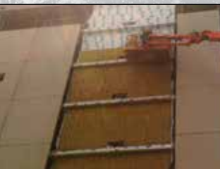
Behind cladding over concrete block walls
