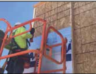
Behind cladding over wood stud walls
