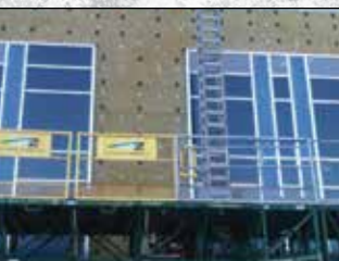
Behind cladding over steel stud walls
