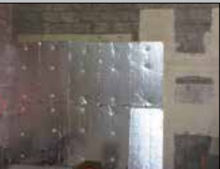
Interior walls on concrete block
