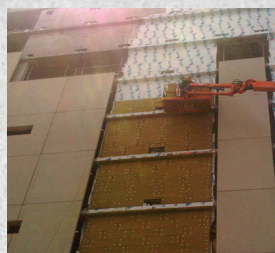
Behind cladding over concrete block walls
