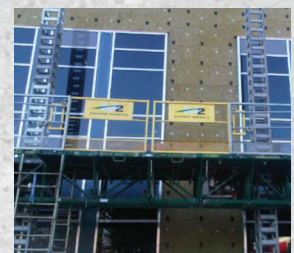
Behind cladding over steel stud walls
