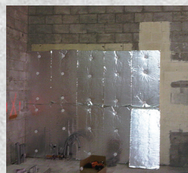
Interior walls on concrete block
