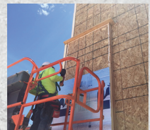
Behind cladding over wood stud walls
