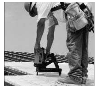
Plywood attachment—using TrakFast plywood to steel pin
