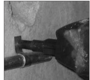
12HSMP034 clip assembly used to secure conduit
