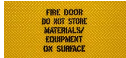
YB - Door painted yellow with "FIRE DOOR DO NOT STORE MATERIALS/EQUIPMENT ON SURFACE" in black lettering (Not available on AR cover)
