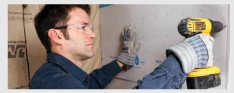
**NOTE:** Make sure your fasteners are flush with the surface of the GoBoard.
