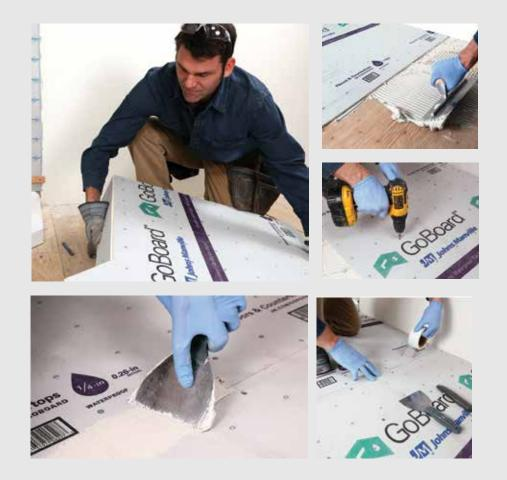
NOTE: Be sure to follow the manufacturer's instructions when mixing and applying the mortar. NOTE: Stagger all board joints to make sure they do not line up with the subfloor joints. NOTE: Skip the fastening step if you are installing on concrete floors.
