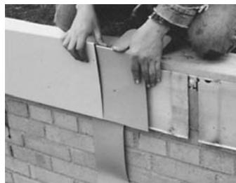
JM PVC-Coated Metal is a special flashing material used to fasten some JM PVC Membranes at roof edges (perimeters), walls and decks, and around penetrations. It is supplied in large, galvanized sheets with JM PVC Membrane material laminated to one side. The roof membrane is welded to this surface. The other side is covered with a protective coating (bronze color).
