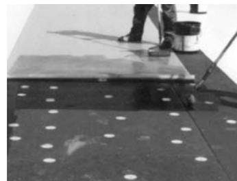
When using mechanical fasteners, if you are unsure of the deck condition, perform pull-out tests of the fasteners being used to confirm sufficient pull-out strength. Contact your supervisor, who will obtain full details from the JM Roofing Services Group.
