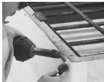
Install all membrane flashings at the same time as the roof membrane. Do not use temporary flashings. If water penetrates the flashings, immediately replace all affected materials.
