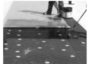
When using mechanical fasteners, if you are unsure of the deck condition, perform pull-out tests of the fasteners being used to confirm sufficient pull-out strength. Contact your supervisor, who will obtain full details from the JM Roofing Services Group.
