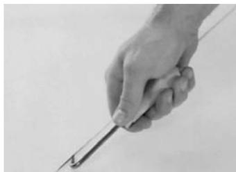
Test all welded seams for integrity and continuity before the end of each work day. In addition to probing, take seam samples to verify seam quality as necessary.
