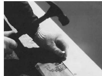
Preformed JM PVC-Coated Metal Flashing is fastened around the roof perimeter (edge and base flashings) and roof penetrations. Welding the membrane to JM PVC-Coated Metal Flashings at these points provides a watertight seal.
