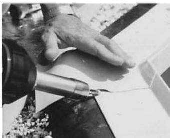
If the vertical gravel stop face exceeds 4" (10.16 cm), fasten per the job specifications, but not less than a 20-gauge to 24-gauge (0.91 mm to 0.61 mm), continuous galvanized steel clip on the fascia.
