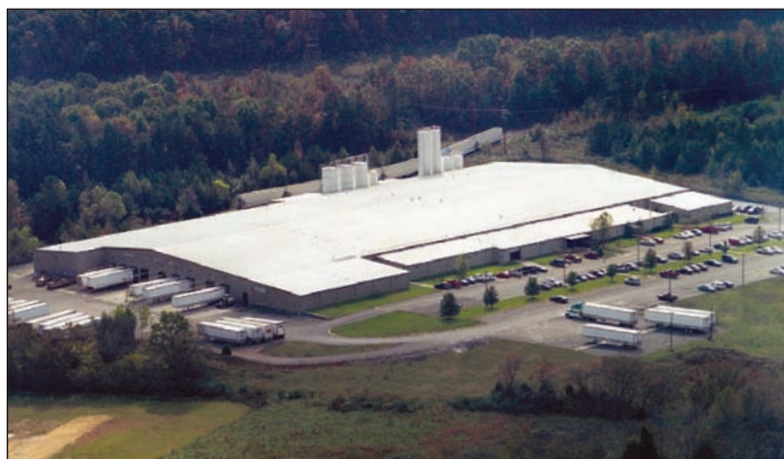
JM TPO manufacturing facility in Scottsboro, Ala.
