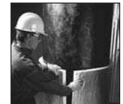
Tank & Equipment Insulation
