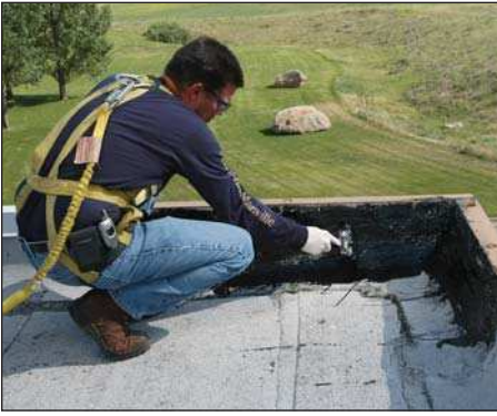
1. Apply base coat
