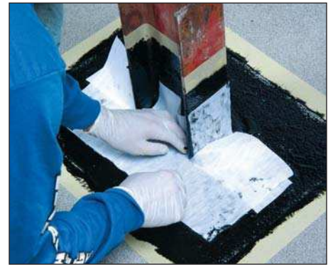
3. Embed PermaFlash Scream
