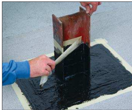
5. Remove masking tape
