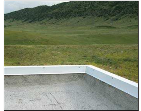
6. Finished wall flashing
