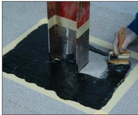
2. Apply base coat
