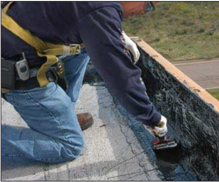
4. Coat entire scrim area
