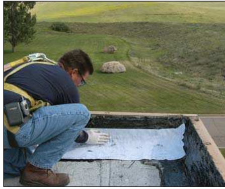
2. Embed PermaFlash Scream
