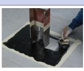
Coat the masked off area with a very thin coating (20-30 mil, 0.51mm-0.76mm) of MBR Flashing Cement. A brush works best.
