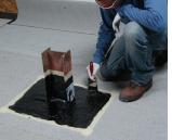
Re-coat the entire masked off area with a thicker (60 mil. 1.52 mm) coating of MBR Flashing Cement.
