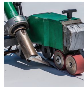
Heat Welding Seams
