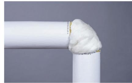
**3.** Butt the ends of the fiber glass insert against the ends of the pipe covering. Tuck and fold the insulation so that it covers all bare surfaces. Keep the fiber glass fluffed up to the thickness of the adjacent pipe insulation to assure maximum thermal efficiency.
