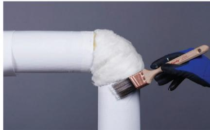
**4.** Apply a vapor barrier mastic around the edges of the adjoining pipe insulation.
