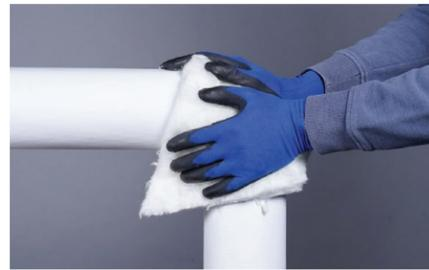
**2.** Place the pre-cut fiber glass insert around the fitting, positioning the points of the insert on the inside radius of the elbow. For applications with temperatures below 45°F (7°C) or above 250°F (121°C), additional layers of insulation may be required.\* In such cases, the first layer is secured by wrapping with fiber glass yarn.
