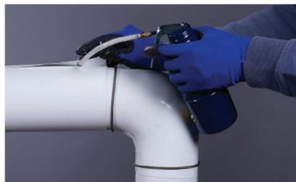
**4.** Overlap the jacketing on itself (approximately 1½" to 2" [38 mm to 51 mm]) and apply a bead of adhesive along the entire length of the longitudinal lap. Place elastic cords or PVC tape around the jacketing.
