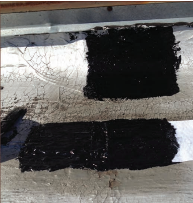
Karna-Flex 3-course repair on asphalt BUR with aged aluminum coating.
