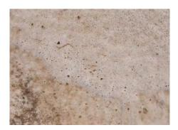
Saturated or wet insulation– Leads to loss of R-value
