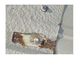
Accelerated deterioration of roof surface
