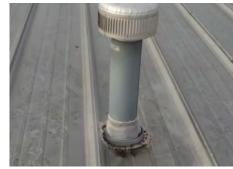
Leaks into interior of structure
