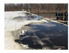
Membrane deterioration–which can lead to premature failure of roof
