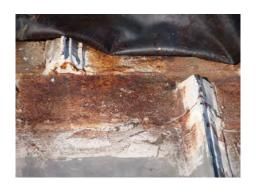
When rust is this bad, KARNAK products will not work to repair; the panel must be replaced so a roofing professional must be contacted.
