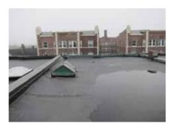
Membrane deteriorationwhich can lead to premature failure of roof
