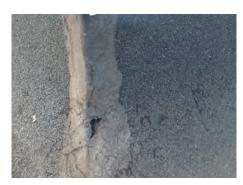
Water leaks into roof systemcan lead to mold and rot Saturated or wet insulation-
