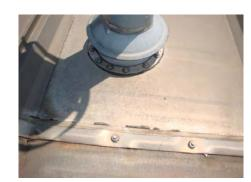
Leaks into interior of structure
