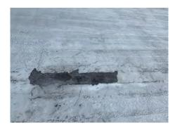
Asphalt deterioration—which can lead to premature failure of roof
