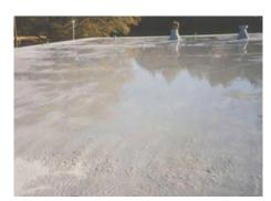
Membrane deteriorationwhich can lead to premature failure of roof rot
