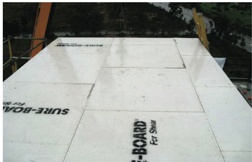
Sure-Board Series 200S is the non-combustible alternative for any CFS® sheathing application both large and small.
