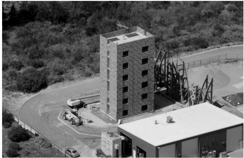
Sure-Board was put to the "Real Test" at the world's largest outdoor shake table at UCSD.
