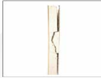
Rigid plastic wall panel Complete structural failure
