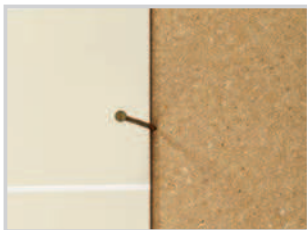
Place a 6 penny spacing nail between panels.
