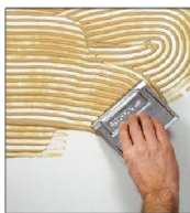
Apply Marlite Brand Adhesive to the back of panels and apply to a subwall.
