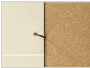
Place a 6 penny spacing nail between panels.
