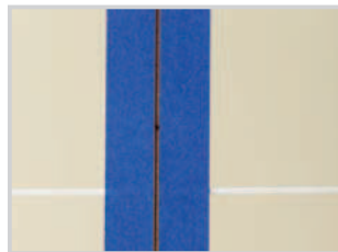
After adhesive dries one hour, remove nail and protect face with tape.
