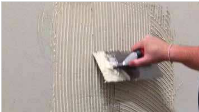
Apply Marlite adhesive evenly to the wall using a trowel.
