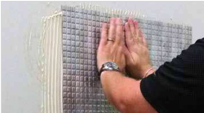
Press the panel against the wall.
