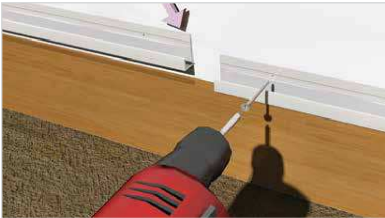
Attach the CP-280 Edge at bottom of installation and perimeter trim.
