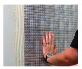
Apply pressure evenly on the different parts of the panel to ensure adhesion.
