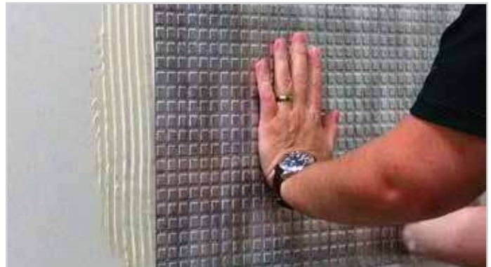
Apply pressure evenly on different parts of the panel to ensure adhesion.
