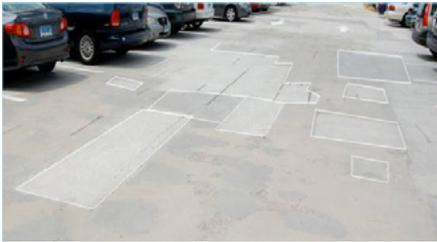
Figure 10 – Incipient Anode Effect on Parking Structure
