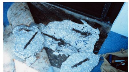
Figure 8 – Corrosion Induced Failure Following Application of a Deck Membrane
