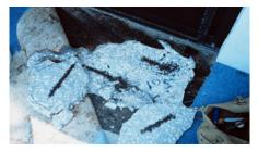
Figure 8 – Corrosion Induced Failure Following Application of a Deck Membrane
