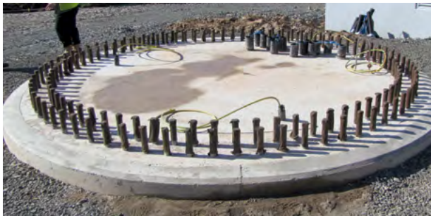
Concrete foundation ready to install turbine
