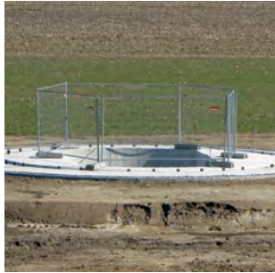
Concrete tower foundation
