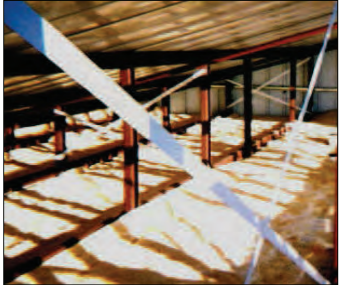
Photo 2 – Unfaced Fiberglass installed over existing roof
