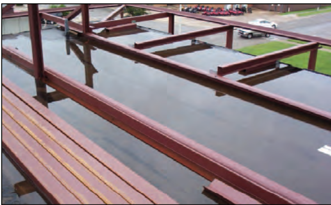
Flooded roof due to continuous members damming rainwater by not having shims installed beneath them
