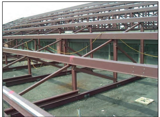
Photo 1 – Retro-Master framing system under construction
