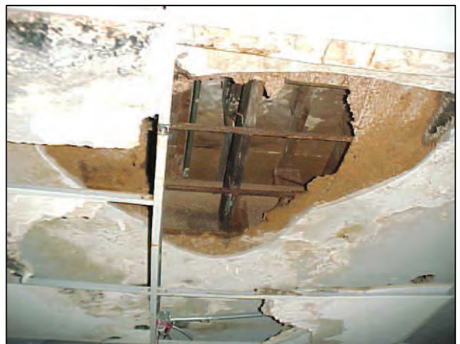
Deteriorated ceiling and exposed wood framed roof support system
