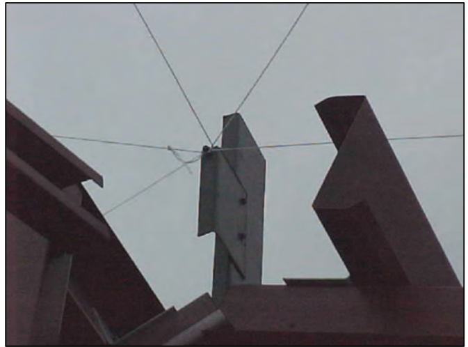
Photo 1 – String Lines Installed at the Intersection of a Hip and Ridge
