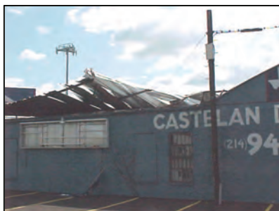
Failed retrofit roof system
