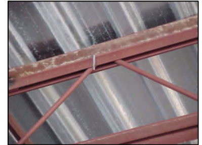
Existing Bar Joist
