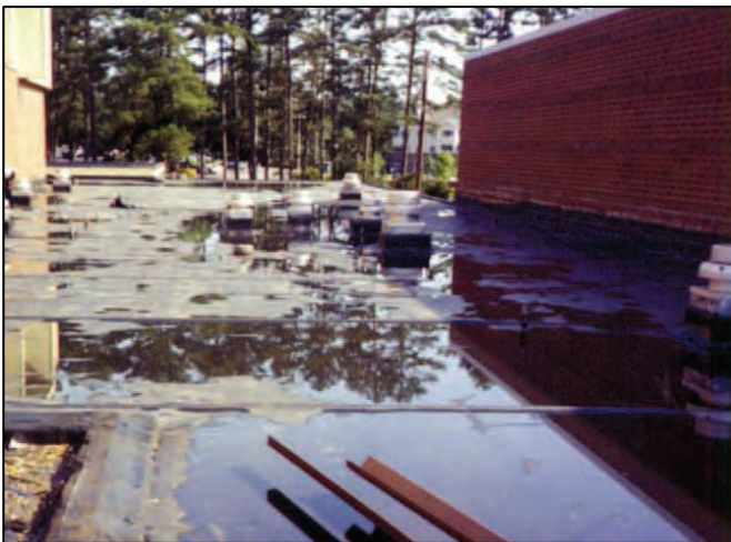
Photo 1 – Ponding water on flat roof
