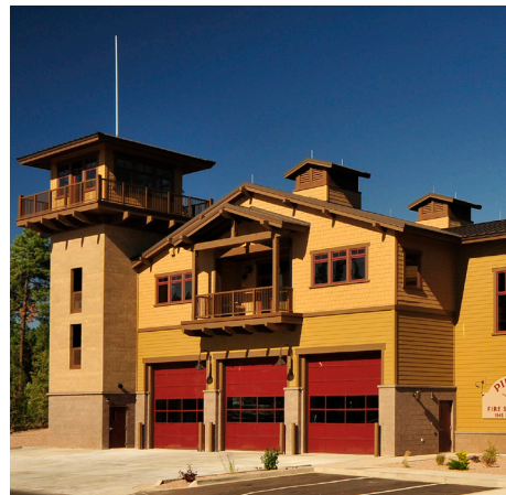
Pinetop Fire Station, Pinetop, AZ
