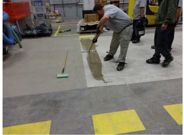
Applying AH HDR Primer with rubber squeegee
