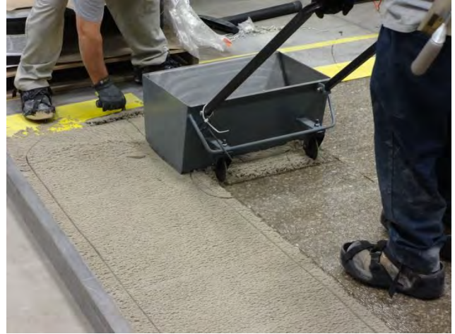
Dropping AH HDR out of the screed box
