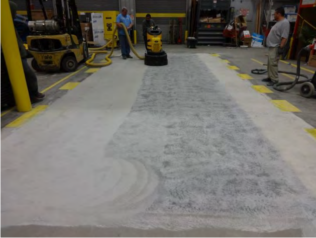
Grinding AH HDR next morning
