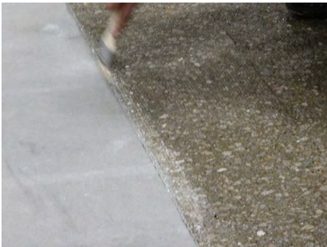
Brush application to get the edges that squeegee couldn't
