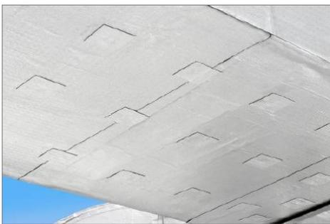
On ducts over 24" (60cm) wide, pin bottom 12" (30cm) on-center. Cover pins with a minimum piece of 3" (7cm) squares of FlexClad® to seal pins from weather.
