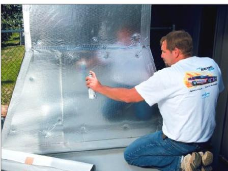
It can also be applied at overlap areas for improved adhesion. Apply a light coat direct to the substrate and wait 2-3 minutes, depending on humidity and wind conditions, or until surface no longer looks wet.
